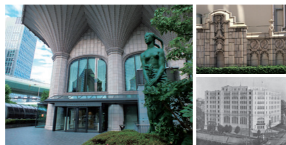
7: 大同生命大阪本社ビル(旧 大同生命肥後橋ビル) | 1993 Daido Life Insurance Osaka Headquarters Building (former Daido Life Insurance Higobashi Building)
