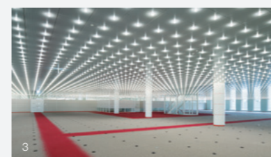
基準階オフィス。放射空調と明るさ照明を組み込んだパンチングメタルの天井を開発した。Standard floor office. The all-over punched metal ceiling was specially developed to incorporate radiant air conditioning and brightness enhancing illumination units.
