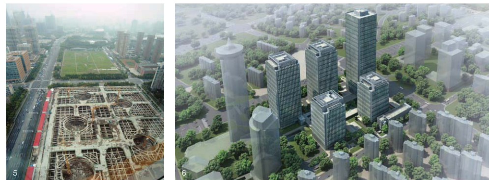
5,6: 塘东中块总部基地項目の現場写真および全景イメージ。事業者の要望を整理し、設計チームとの橋渡しとなるプロジェクト運営を進めている。 5,6: Photograph showing the construction site of the Tangdong Middle Area Headquarters Basic Project, and an overall image. We organize the client's needs and serve as a bridge between the client and the team of designers.
